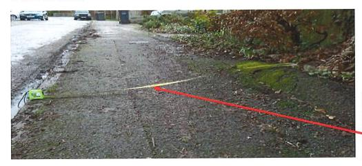
As you can see from the bend in the tape measure the lifting of the pavement starts approximately in the middle of the pavement. Credit:
